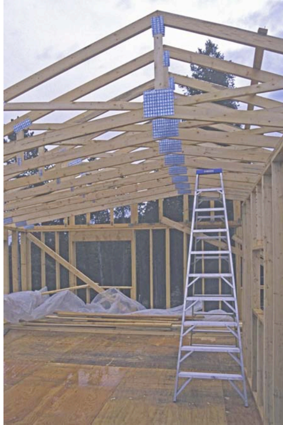
A 10 ft Step Ladder is Needed for Vaulted Ceilings to Reach Roof Trusses and Secure Them with a Temporary 2x4. Note that the thick plywood floor is wet with recent rainfall. If it was an OSB floor, it would be warped with the rain.
