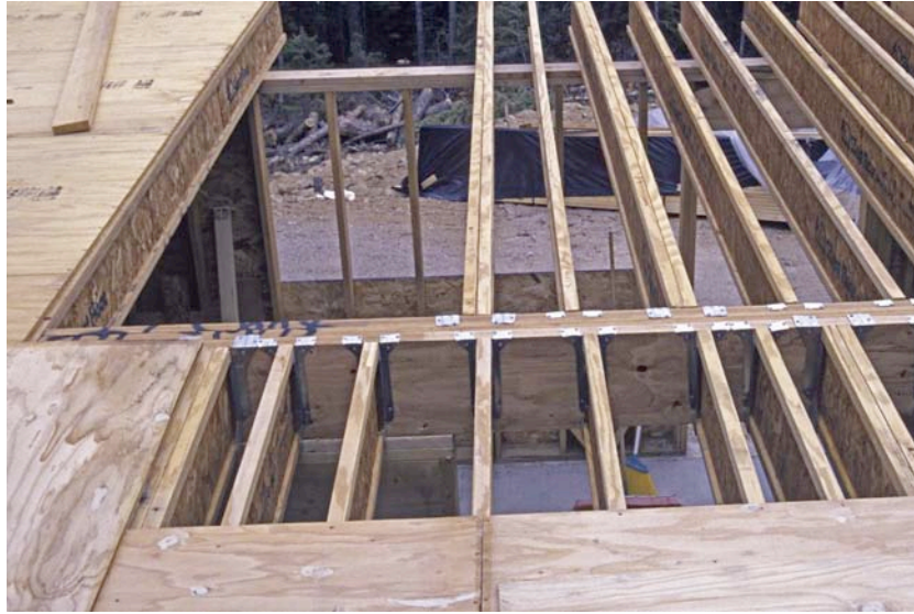
TJI Floor Trusses Installed
