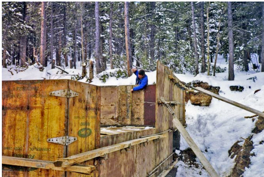
Forms for Pouring the Colorado Foundation Wall on the Footers (Back Wall is 4 ft High). Don't forget to put rigid insulation on the outside of the wall that will be below ground level, and seal the wall with black tar on areas that will be below ground level and above floor level.
