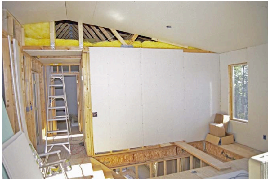
Drywall Installation
