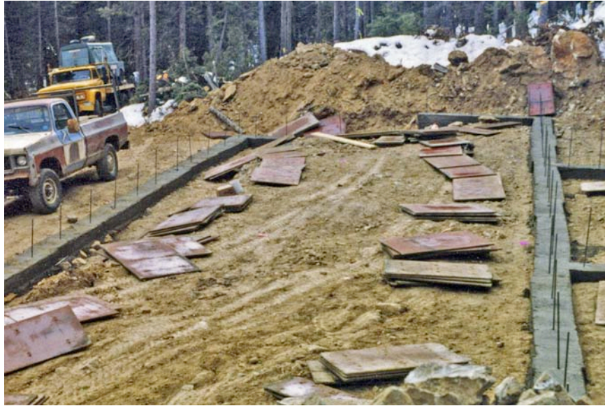
Footers for the Foundation Wall. These do not need to be straight and level like the subsequent foundation wall.
