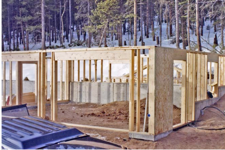
Start of Framing for a “Garage” Home.
