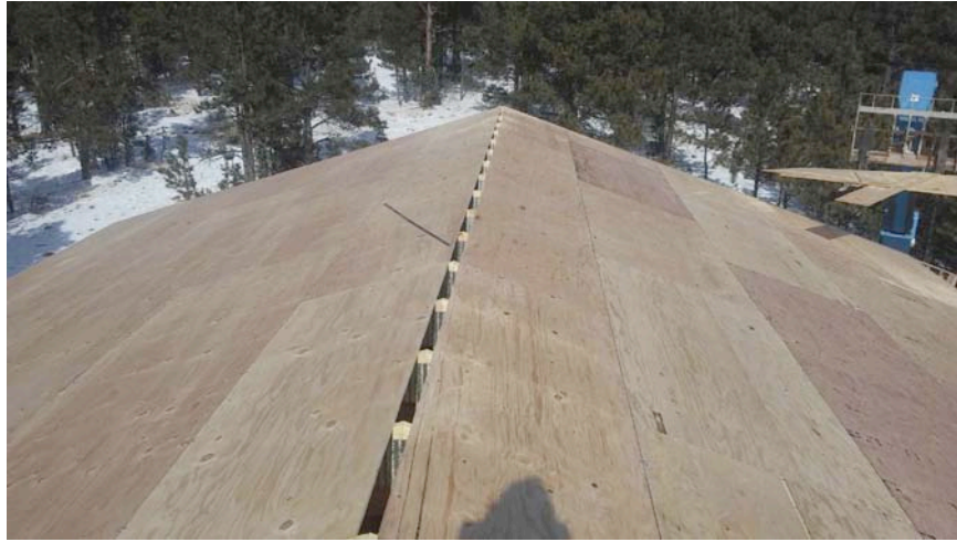
Leave an Opening or Slit the Ridge if Using Roof Ridge Vents. Better to not let a roofing contractor do this step.
